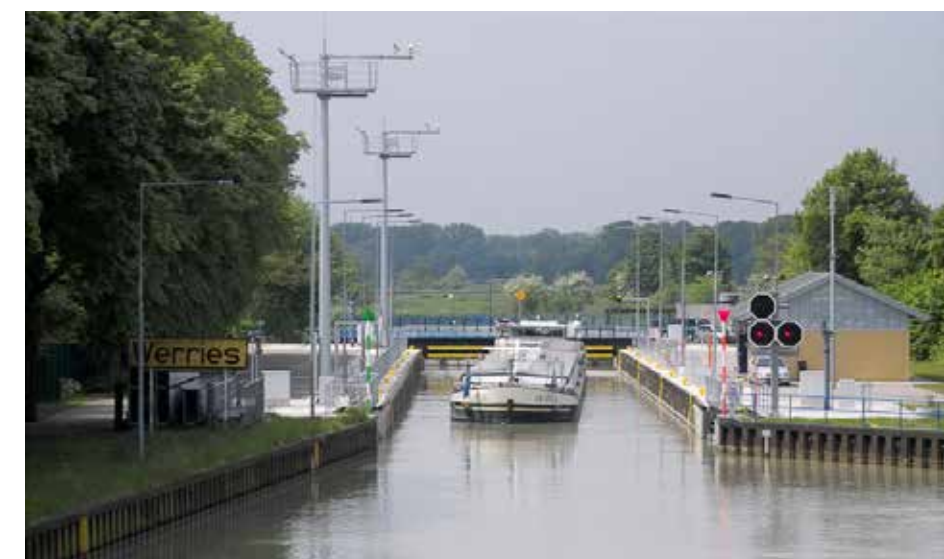
Schleuse Werries. Foto: RIK/Walter
